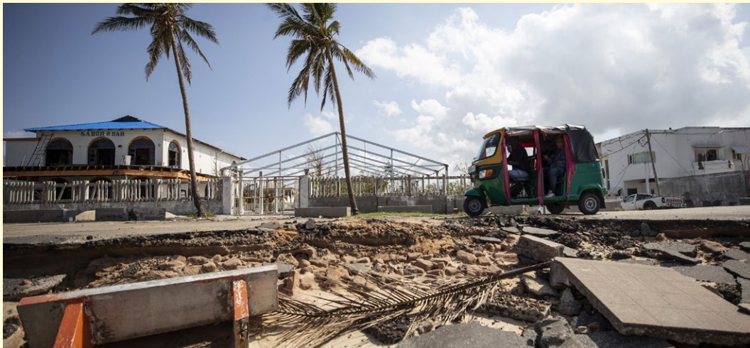
Damaged road is seen following the Cyclone Idai in Sofala region in Beira, Mozambique on March 31, 2019. © Gokhan Balci/Anadolu Agency/Getty Images
