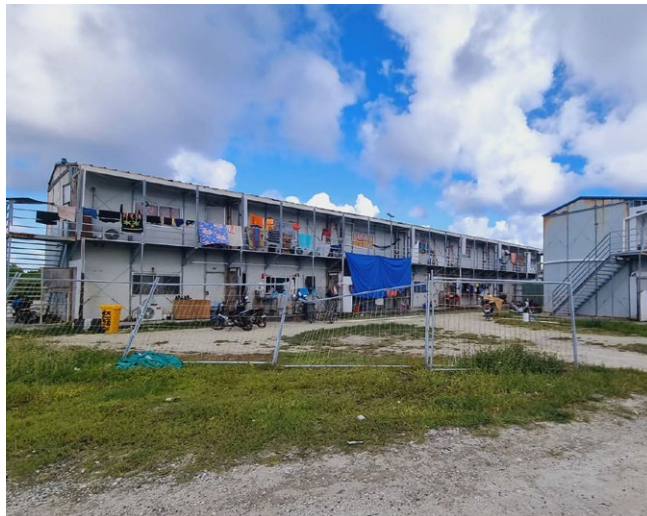
Prefabricated accommodations used to host media during the 2019 Pacific Island Forum converted into housing in Funafuti, Tuvalu. © Amnesty International
